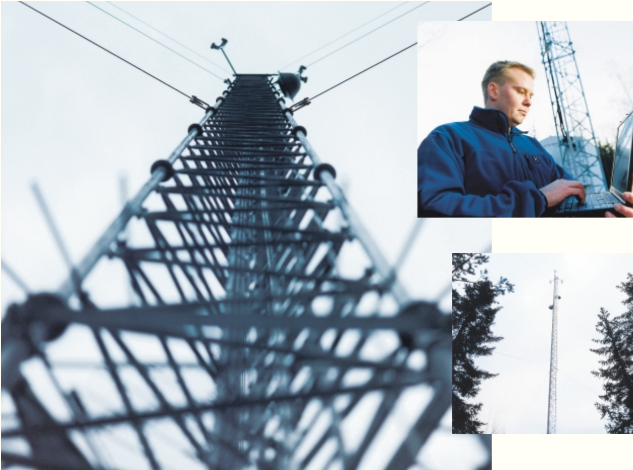
Building infrastructure for the mobile telephony of the future requires strong alliances. NCC has concluded a partnership with Ericsson regarding the build-out of 3G networks.
