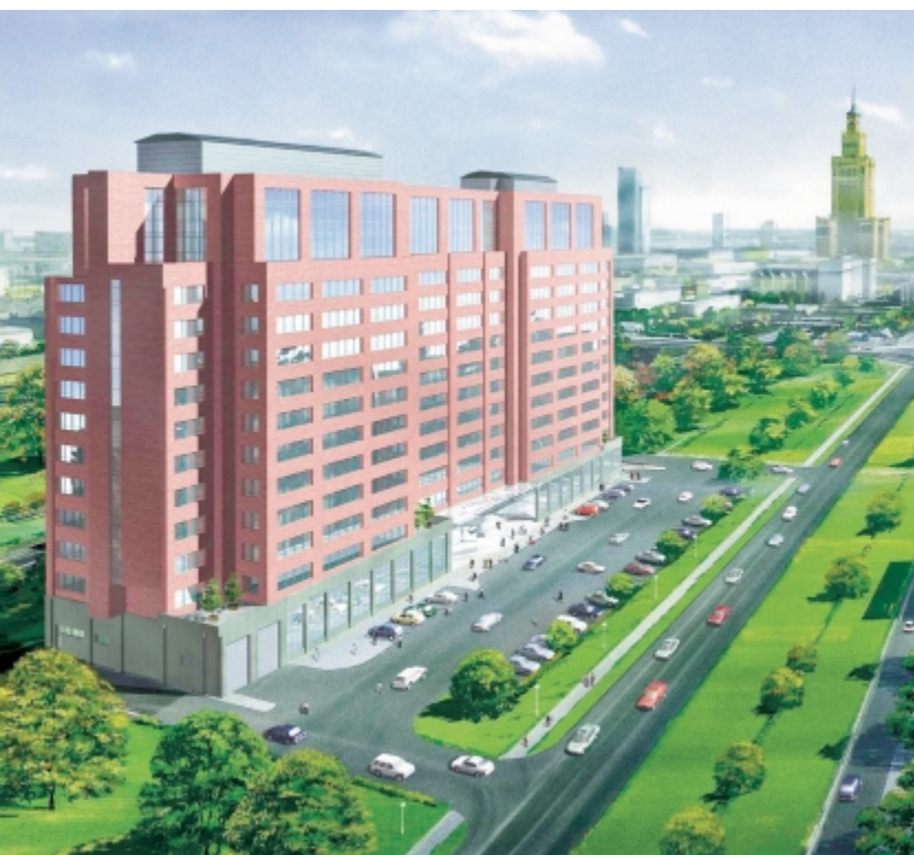
NCC Property Development has projects in progress in such cities as Warsaw.
