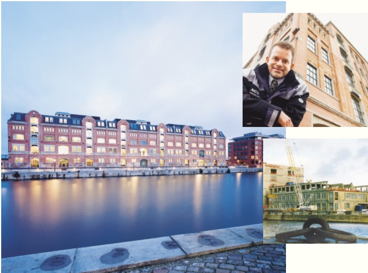
NCC's meticulous renovation of Dahlerups Pakhus in Copenhagen is an award-winning project. Langelinie is currently one of the most attractive locations in Denmark's capital.
