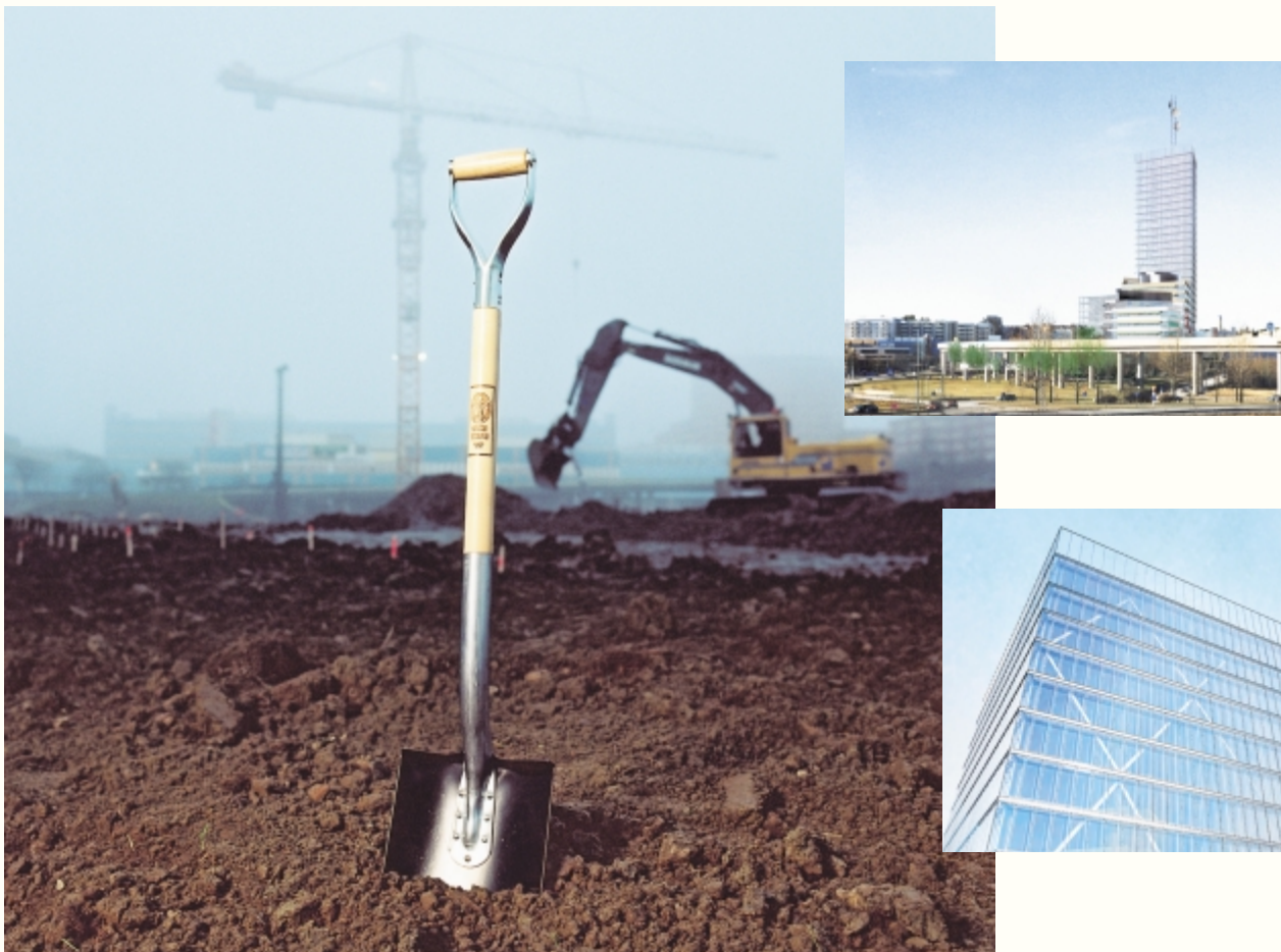
In Kista, NCC is building what will become a symbol for the information society, as well as a new landmark in Stockholm.
